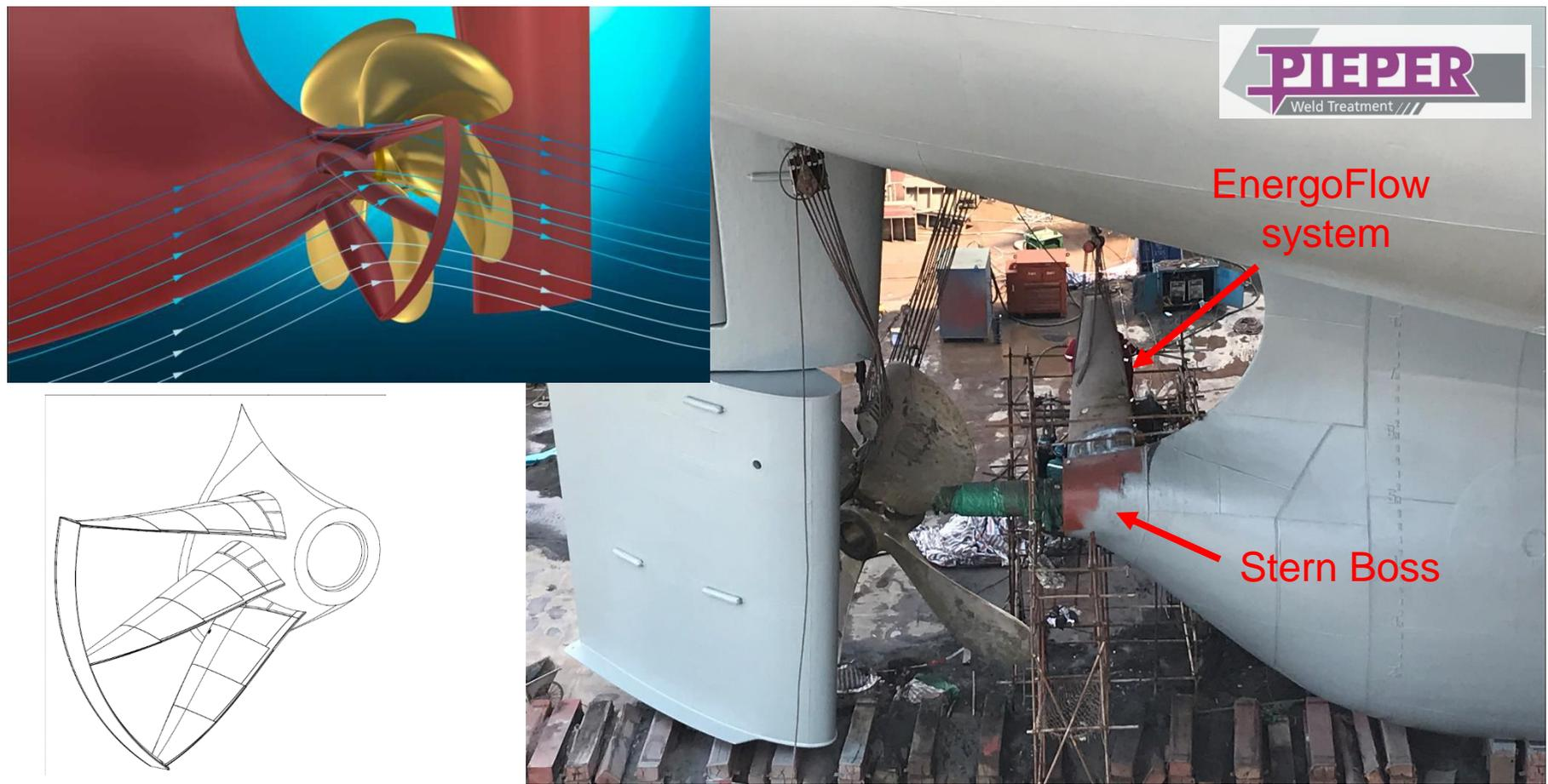
Length of the separate blades is approximately 4000 mm. Due to the dynamic load caused by the water flow, welds will be sensitive to fatigue. HFMI treatment procedure has been drawn up in order to enhance fatigue strength of the critical weld connections. Procedure will be used World Wide for treatment of EnergoFlow systems during installation. (pictures Bulk Carrier MV Cancun treated in Dry-dock Shanghai - China)
